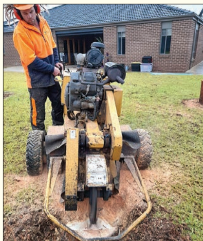
Stump grinding flat, underground or totally remove
