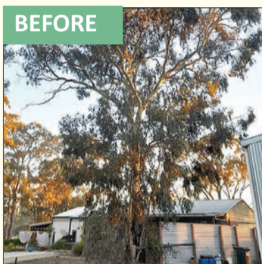
BEFORE This tree re-grew from an old stump and had limbs touching the roof and in amongst the ariel.
